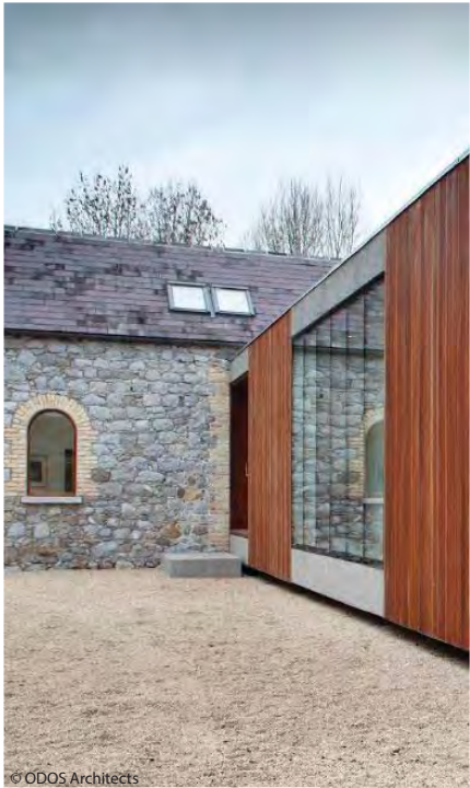
© ODOS Architects Ballymahon, by ODOS Architects
