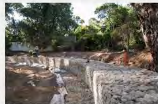
Brownhill Creek Upgrade JWS Morris Gabions January 2019
